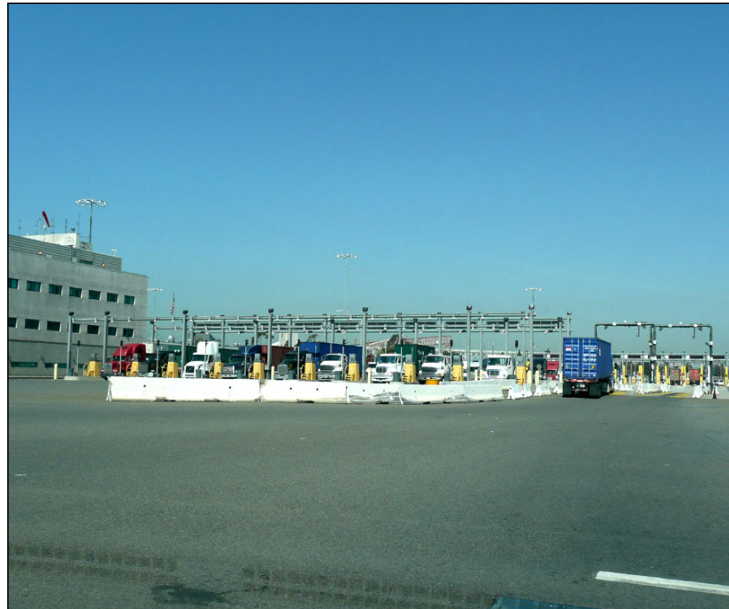
Photograph 7: Existing in-gate and out-gate
