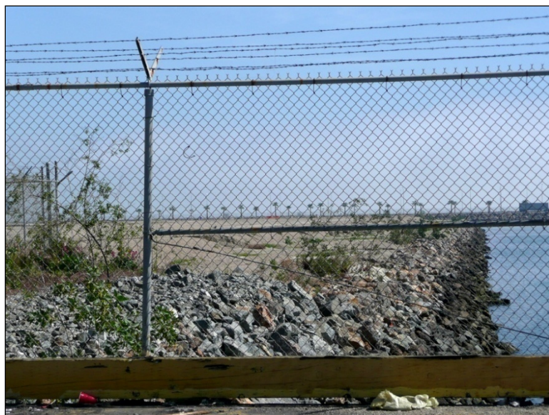
20 21 Photograph 2: Area of new wharf along Berth 306
