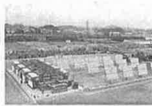
Integrated 1 MW solar photovoltaic and battery storage system (terminal functions as a green microgrid)
