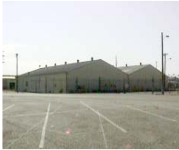
Shed warehouses and parking lots in north end of project site
