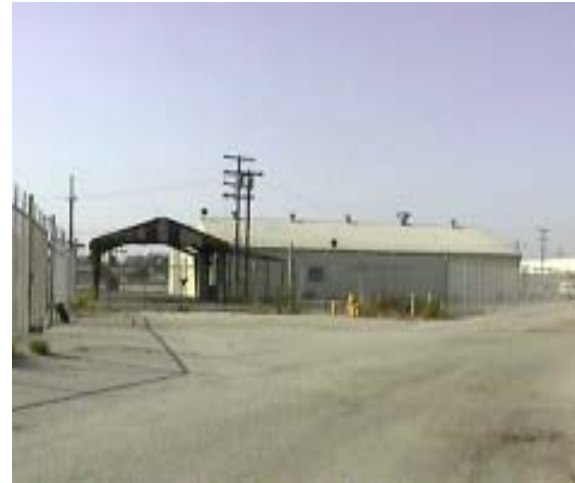
Warehouse and parking lot in northern project site
