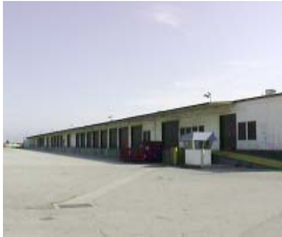
Warehouse No. 6 in northern end of project site at 22nd Street
